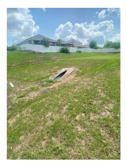
Location 23: Mitered End Sections (MES). MES is showing signs of erosion and is being undermined. Erosion observed beneath existing mitered end section. Add #57 stone with compacted fill beneath eroded areas mitered end section to prevent future erosion and undermining. Place filter fabric and rip rap extending 2' minimum out from existing structure to stabilize the area around the existing mitered end section. Sod disturbed areas.
