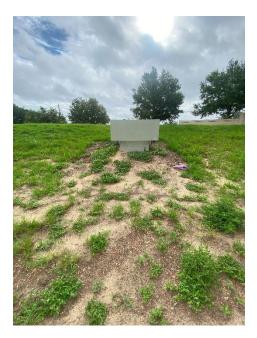
**Location 2:** Silt build up at end of Mitered End Section (MES). Rip rap placed at end of the MES is higher in elevation than the end of the MES. The Rip rap is to be removed and reinstalled with filter fabric and 2' depth of rip rap extending 10' from end of MES to prevent erosion and provide a discharge at or below the invert.
