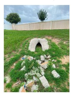
**Location 14:** Silt build up at end of Mitered End Section (MES). Rip rap placed at end of the MES is higher in elevation than the end of the MES restricting flow. The Rip rap is to be removed and reinstalled with filter fabric and 2' depth of rip rap extending 10' from end of MES to prevent erosion and provide a discharge at or below the invert.
