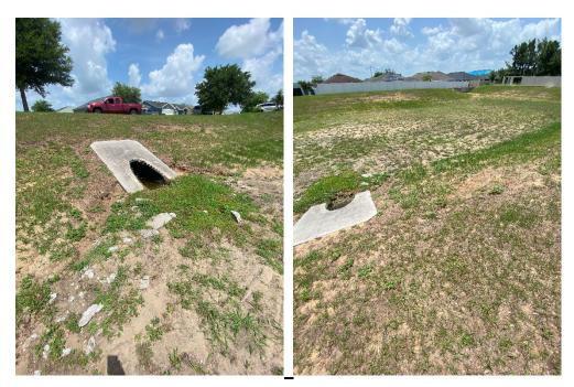
**Location 33:** Silt build up at end of Mitered End Section (MES). Remove silt from end of pipe and determine if additional jetting is required or if the build up of silt is contained at the end of the pipe. Rip rap placed at end of the MES is higher in elevation than the end of the MES. The Rip rap is to be removed and reinstalled with filter fabric and 2' depth of rip rap extending 10' from end of MES to prevent erosion and provide a discharge at or below the invert.
