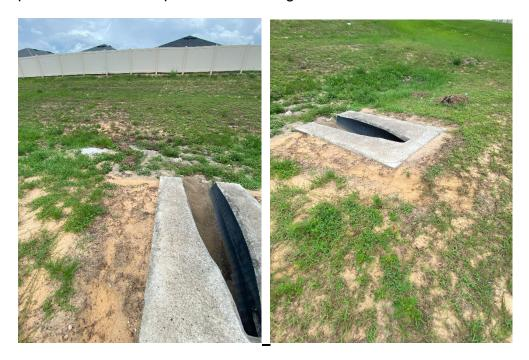
Location 10: Silt build up at end of Mitered End Section (MES). Remove silt from end of pipe and determine if additional jetting is required or if the build up of silt is contained at the end of the pipe. Rip rap placed at end of the MES has been displaced.. The Rip rap is to be removed and reinstalled with filter fabric and 2' depth of rip rap extending 10' from end of MES to prevent erosion and provide a discharge at or below the invert.
