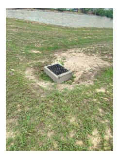
**Location 18:** Silt build up at end of Mitered End Section (MES). Remove silt from end of pipe and determine if additional jetting is required or if the build up of silt is contained at the end of the pipe. Rip rap placed at end of the MES has been displaced.. The Rip rap is to be removed and reinstalled with filter fabric and 2' depth of rip rap extending 10' from end of MES to prevent erosion and provide a discharge at or below the invert.
