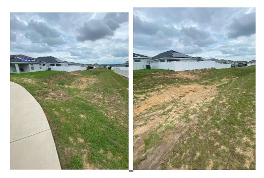
**Location 13:** Silt build up at end of Mitered End Section (MES). Remove silt from end of pipe and determine if additional jetting is required or if the build up of silt is contained at the end of the pipe. Rip rap placed at end of the MES has been displaced.. The Rip rap is to be removed and reinstalled with filter fabric and 2' depth of rip rap extending 10' from end of MES to prevent erosion and provide a discharge at or below the invert.
