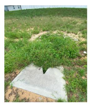
**Location 19:** Silt build up at end of Mitered End Section (MES). Remove silt from end of pipe and determine if additional jetting is required or if the build up of silt is contained at the end of the pipe. Rip rap placed at end of the MES has been displaced.. The Rip rap is to be removed and reinstalled with filter fabric and 2' depth of rip rap extending 10' from end of MES to prevent erosion and provide a discharge at or below the invert.
