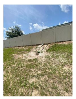
**Location 31:** Silt build up at end of Mitered End Section (MES). Remove silt from end of pipe and determine if additional jetting is required or if the build up of silt is contained at the end of the pipe. Rip rap placed at end of the MES is higher in elevation than the end of the MES. The Rip rap is to be removed and reinstalled with filter fabric and 2' depth of rip rap extending 10' from end of MES to prevent erosion and provide a discharge at or below the invert.
