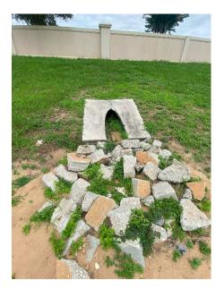
Location 16: Remove obstruction and silt from discharge pipe. Place rip rap 5' from outfall.
