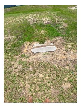
**Location 32:** Lack of turff makes the area susceptible to erosion. Review during rainy season for additional growth. If turf does not reestablish itself, we recommend placing sod in area. Remove silt and debris from end of pipe.
