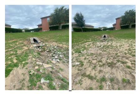
Location 8: Lack of turff makes the area susceptible to erosion. Review during rainy season to determine if turf will re-estblish. Re-evaluate in 60 days.
