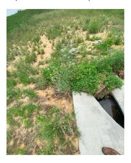
Location 20: Silt build up at end of Mitered End Section (MES). Remove silt from end of pipe and determine if additional jetting is required or if the build up of silt is contained at the end of the pipe. Rip rap placed at end of the MES has been displaced.. The Rip rap is to be removed and reinstalled with filter fabric and 2' depth of rip rap extending 10' from end of MES to prevent erosion and provide a discharge at or below the invert.
