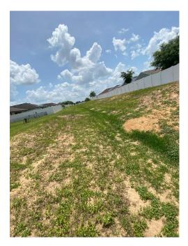
**Location 29:** Lack of turff makes the area susceptible to erosion. Review during rainy season for additional growth. If turf does not reestablish itself, we recommend placing sod in area.
