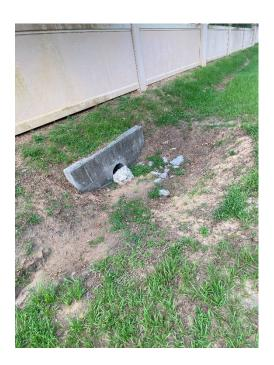
Location 17: Silt build up at end of Mitered End Section (MES). Remove silt from end of pipe and determine if additional jetting is required or if the build up of silt is contained at the end of the pipe. Rip rap placed at end of the MES is higher in elevation than the end of the MES. The Rip rap is to be removed and reinstalled with filter fabric and 2' depth of rip rap extending 10' from end of MES to prevent erosion and provide a discharge at or below the invert.
