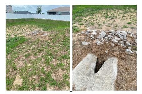
**Location 8:** Silt build up at end of Mitered End Section (MES). Rip rap placed at end of the MES is higher in elevation than the end of the MES. The Rip rap is to be removed and reinstalled with filter fabric and 2' depth of rip rap extending 10' from end of MES to prevent erosion and provide a discharge at or below the invert.
