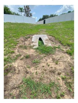
Location 21: Swale bottom eroding. Regrade and sod all disturbed areas.
