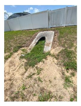
**Location 36:** Erosion at discharge pipe. Place rip rap with filter fabric extending 10' from Mitered End Section.
