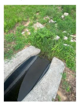
**Location 10:** Silt build up at end of Mitered End Section (MES). Rip rap placed at end of the MES is higher in elevation than the end of the MES. The Rip rap is to be removed and reinstalled with filter fabric and 2' depth of rip rap extending 10' from end of MES to prevent erosion and provide a discharge at or below the invert. Place rip rap 2' around MES to prevent future erosion and undermining.
