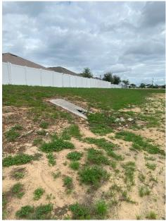
**Location 4:** Erosion due to resident construction. Verify this area is restored to original condition after construction is completed.
