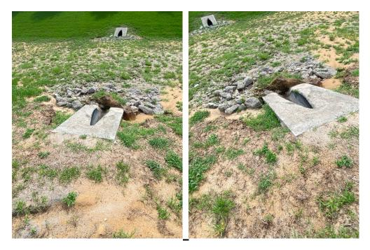
**Location 11:** Erosion at end of Mitered End Section (MES). The Rip rap is to be removed and reinstalled with filter fabric and 2' depth of rip rap extending 10' from end of MES to prevent erosion and provide a discharge at or below the invert.
