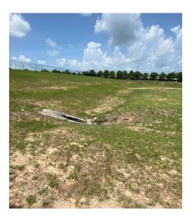
**Location 37:** Lack of turff makes the area susceptible to erosion. Review during rainy season for additional growth. If turf does not reestablish itself, we recommend placing sod in area.
