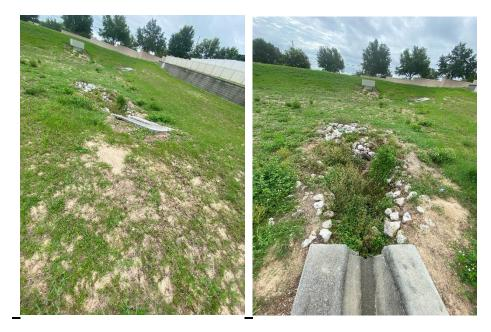
**Location 4:** Lack of turff makes the area susceptible to erosion. Review during rainy season for additional growth. If turf does not reestablish itself, we recommend placing sod in area or seeding the area encourace growth.
