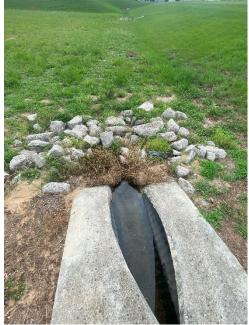
**Location 9:** Remove silt and vegetation from end of pipe to below invert. Place rip rap with filter fabric extending 5' from end of pipe. Rip rap is to be placed below invert to allow flow.
