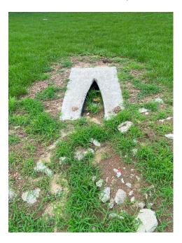
**Location 13:** Silt build up at end of Mitered End Section (MES). Remove silt from end of pipe and determine if additional jetting is required or if the build up of silt is contained at the end of the pipe. Rip rap placed at end of the MES is higher in elevation than the end of the MES. The Rip rap is to be removed and reinstalled with filter fabric and 2' depth of rip rap extending 10' from end of MES to prevent erosion and provide a discharge at or below the invert.
