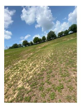
**Location 40:** Lack of turff makes the area susceptible to erosion. Review during rainy season for additional growth. If turf does not reestablish itself, we recommend placing sod in area.
