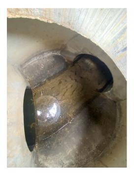
**Location 3:** Silt build up at end of Mitered End Section (MES). Rip rap placed at end of the MES is higher in elevation than the end of the MES. The Rip rap is to be removed and reinstalled with filter fabric and 2' depth of rip rap extending 10' from end of MES to prevent erosion and provide a discharge at or below the invert.
