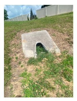
**Location 26:** Silt build up at end of Mitered End Section (MES). Remove silt from end of pipe and determine if additional jetting is required or if the build up of silt is contained at the end of the pipe. Rip rap placed at end of the MES is higher in elevation than the end of the MES. The Rip rap is to be removed and reinstalled with filter fabric and 2' depth of rip rap extending 10' from end of MES to prevent erosion and provide a discharge at or below the invert.
