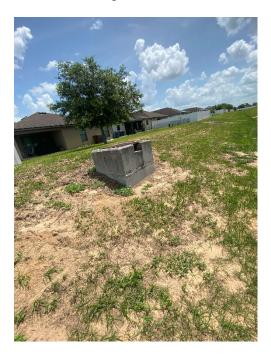
**Location 30:** Pipe extending from residents property causing erosion. Recommend sending a letter to the homeowner requesting they do not discharge into a CDD drainage area and restore the area back to the original condition.
