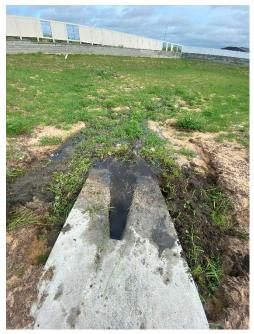
**Location 6:** Lack of turff makes the area susceptible to erosion. Review during rainy season for additional growth. If turf does not reestablish itself, we recommend placing sod in area.
