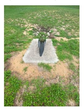
**Location 15:** Silt build up at end of Mitered End Section (MES). Rip rap placed at end of the MES is higher in elevation than the end of the MES restricting flow. The Rip rap is to be removed and reinstalled with filter fabric and 2' depth of rip rap extending 10' from end of MES to prevent erosion and provide a discharge at or below the invert.
