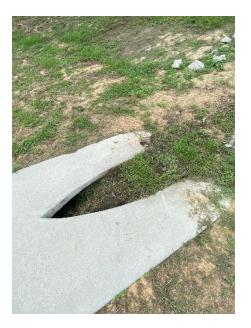
**Location 14:** Silt build up at end of Mitered End Section (MES). Rip rap placed at end of the MES is higher in elevation than the end of the MES restricting flow. The Rip rap is to be removed and reinstalled with filter fabric and 2' depth of rip rap extending to other existing MES to deter erosion.
