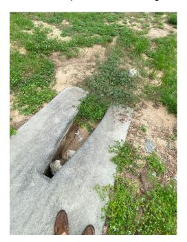
Location 3: Mitered End Sections (MES). MES is showing signs of erosion and is being undermined. Erosion observed beneath existing mitered end section. Add #57 stone with compacted fill beneath eroded areas mitered end section to prevent future erosion and undermining. Place filter fabric and rip rap extending 2' minimum out from existing structure to stabilize the area around the existing mitered end section. Sod disturbed areas.
