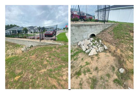
Location 17: Lack of turff makes the area susceptible to erosion. Review during rainy season to determine if turf will re-estblish. Re-evaluate in 60 days.
