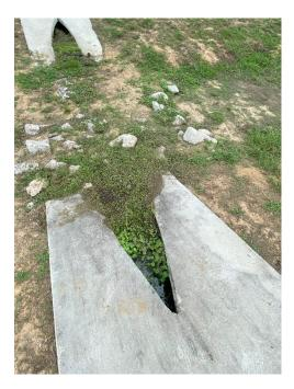
Location 15: Lack of turff makes the area susceptible to erosion. Review during rainy season to determine if turf will re-estblish. Re-evaluate in 60 days.
