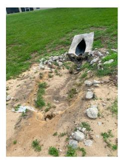
**Location 12:** Silt build up at end of Mitered End Section (MES). Remove silt from end of pipe and determine if additional jetting is required or if the build up of silt is contained at the end of the pipe. Rip rap placed at end of the MES is higher in elevation than the end of the MES. The Rip rap is to be removed and reinstalled with filter fabric and 2' depth of rip rap extending 10' from end of MES to prevent erosion and provide a discharge at or below the invert.
