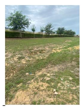
**Location 7:** Discharge slab is eroding. Place fill mixed with #57 stone under slab. Place rip rap with filter fabric 10' from discharge slab
