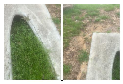
Location 2: Silt build up in structure. Remove silt from structure.
