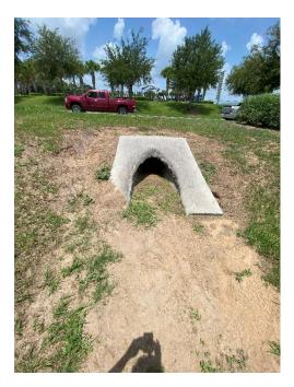
**Location 34:** Lack of turff makes the area susceptible to erosion. Review during rainy season for additional growth. If turf does not reestablish itself, we recommend placing sod in area.
