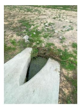
**Location 11:** Silt build up at end of Mitered End Section (MES). Remove silt from end of pipe and determine if additional jetting is required or if the build up of silt is contained at the end of the pipe. Rip rap placed at end of the MES has been displaced.. The Rip rap is to be removed and reinstalled with filter fabric and 2' depth of rip rap extending 10' from end of MES to prevent erosion and provide a discharge at or below the invert.
