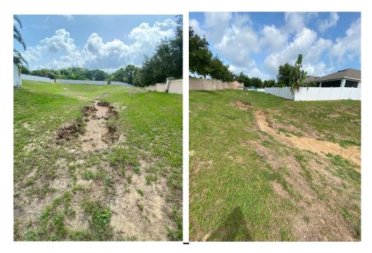
Location 22: Mitered End Sections (MES). MES is showing signs of erosion and is being undermined. Erosion observed beneath existing mitered end section. Add #57 stone with compacted fill beneath eroded areas mitered end section to prevent future erosion and undermining. Place filter fabric and rip rap extending 2' minimum out from existing structure to stabilize the area around the existing mitered end section. Sod disturbed areas.
