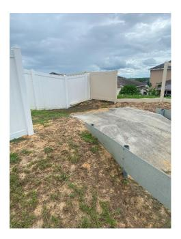
**Location 16:** Remove and replace existing rip rap to be below invert of outflow pipe. Rip rap to extend 10' from outfall point. Clear silt from pipe and evaluate if additional vac and jetting of the pipe is required.
