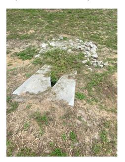
**Location 12:** Lack of turff makes the area susceptible to erosion. Review during rainy season to determine if turf will re-estblish. Re-evaluate in 60 days. Place fill along sidewalk to match the top of the sidewalk grade. Sod all disturbed areas.
