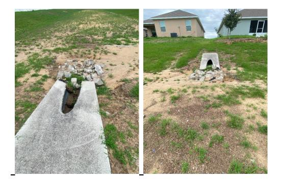
**Location 6:** Lack of turff makes the area susceptible to erosion. Review during rainy season to determine if turf will re-estblish. Re-evaluate in 60 days.
