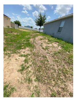
**Location 35:** Silt build up at end of Mitered End Section (MES). Remove silt from end of pipe and determine if additional jetting is required or if the build up of silt is contained at the end of the pipe. Rip rap placed at end of the MES is higher in elevation than the end of the MES. The Rip rap is to be removed and reinstalled with filter fabric and 2' depth of rip rap extending 10' from end of MES to prevent erosion and provide a discharge at or below the invert.
