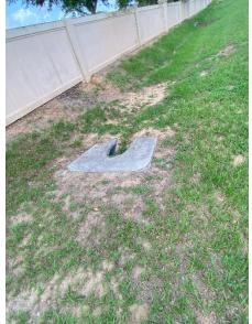
**Location 18:** Silt build up at end of Mitered End Section (MES). Remove silt from end of pipe and determine if additional jetting is required or if the build up of silt is contained at the end of the pipe. Rip rap placed at end of the MES is higher in elevation than the end of the MES. The Rip rap is to be removed and reinstalled with filter fabric and 2' depth of rip rap extending 10' from end of MES to prevent erosion and provide a discharge at or below the invert.
