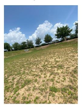
**Location 39:** Lack of turff makes the area susceptible to erosion. Review during rainy season for additional growth. If turf does not reestablish itself, we recommend placing sod in area.
