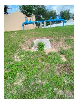
**Location 19:** Lack of turff makes the area susceptible to erosion. Review during rainy season for additional growth. If turf does not reestablish itself, we recommend placing sod in area.
