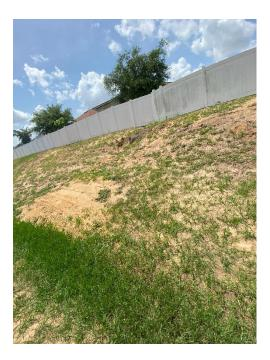
Location 28: Lack of turff makes the area susceptible to erosion. Review during rainy season for additional growth. If turf does not reestablish itself, we recommend placing sod in area.
