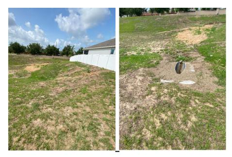
Location 20: Silt build up at end of Mitered End Section (MES). Remove silt from end of pipe and determine if additional jetting is required or if the build up of silt is contained at the end of the pipe. Rip rap placed at end of the MES is higher in elevation than the end of the MES. The Rip rap is to be removed and reinstalled with filter fabric and 2' depth of rip rap extending 10' from end of MES to prevent erosion and provide a discharge at or below the invert.
